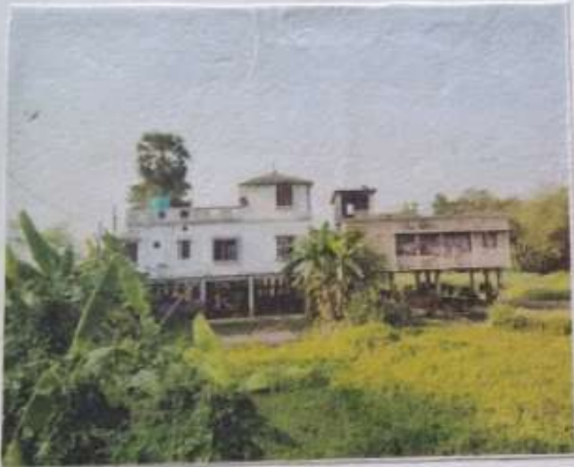
Pic: House types in floodprone area for flood management
