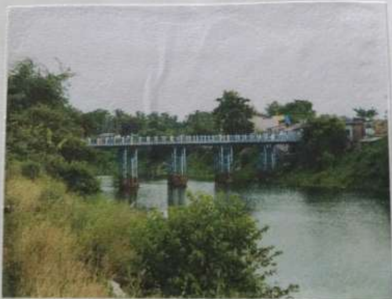
Pic: Local Dam of Daspur-1 block
