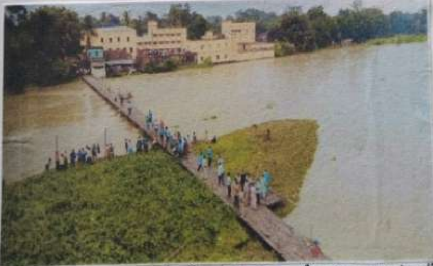
Pic: Wooden Dam in flooded area for communication
