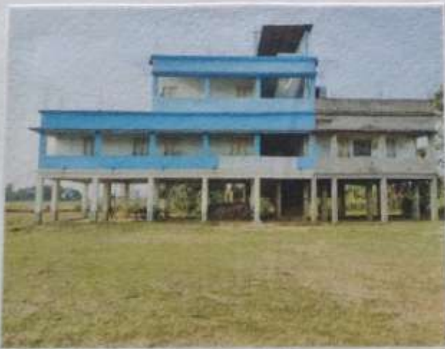
Pic: Upper primary school Building in flood prone area
