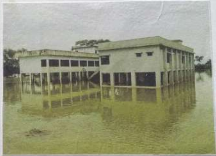
Pic: Houses structure in flooded area
